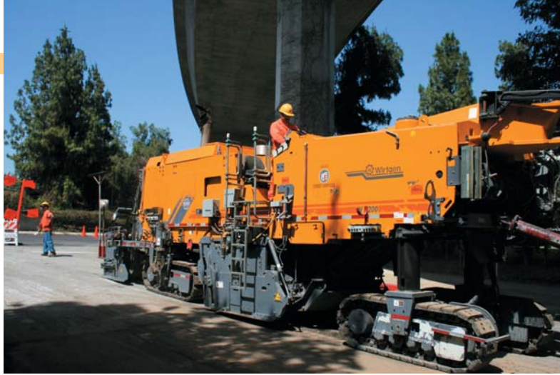
Los Angeles conducts base recycling program prior to overlays using own equipment
